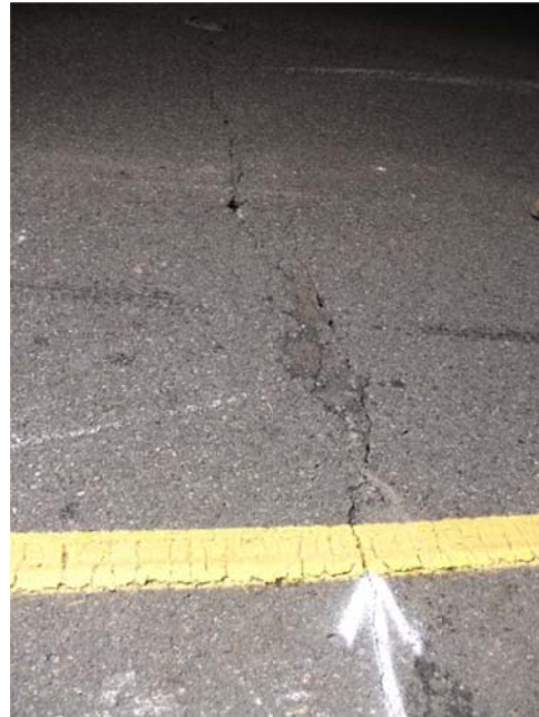
Picture 2. Joint Condition
