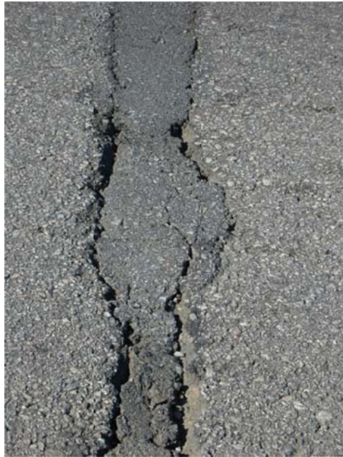
Picture 1. Joint Condition
